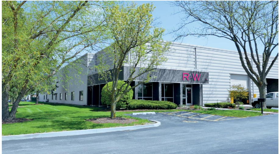
New R+W America Production site in West Chicago, IL
